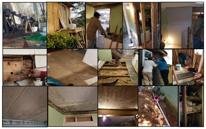
Dangerous back porch, leaking roof in every room, kitchen floor caving in, plumbing repair for bathrooms, no real closets, etc., - Near total house renovation required.
